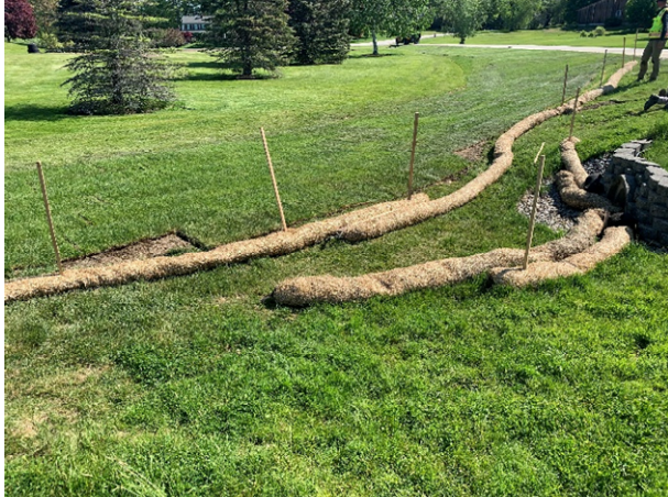
29 Gundalow - 1 (Drainage Area)
