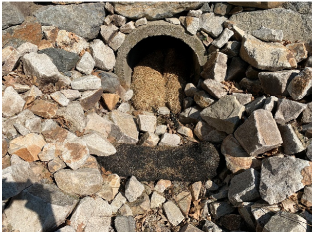
64 Gundalow - 1 (Drainage Course)
