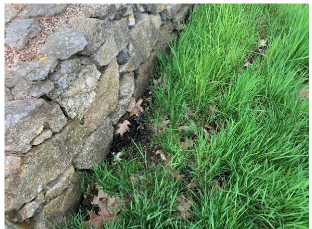
4 Brickyard Circle - 2 (Drainage Course)
