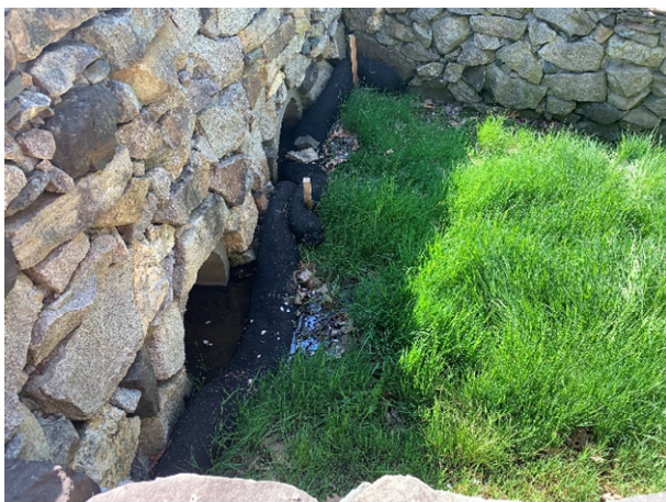
4 Brickyard Circle - 1 (Drainage Course)
